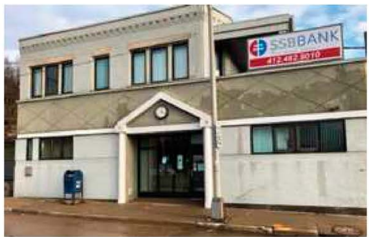
SSB Bank Located in Lower Marshall-Shadeland
